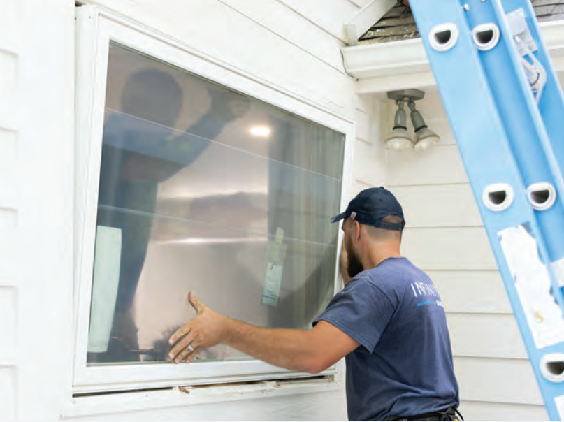
INSTALLATION METHOD: INSERT REPLACEMENT
